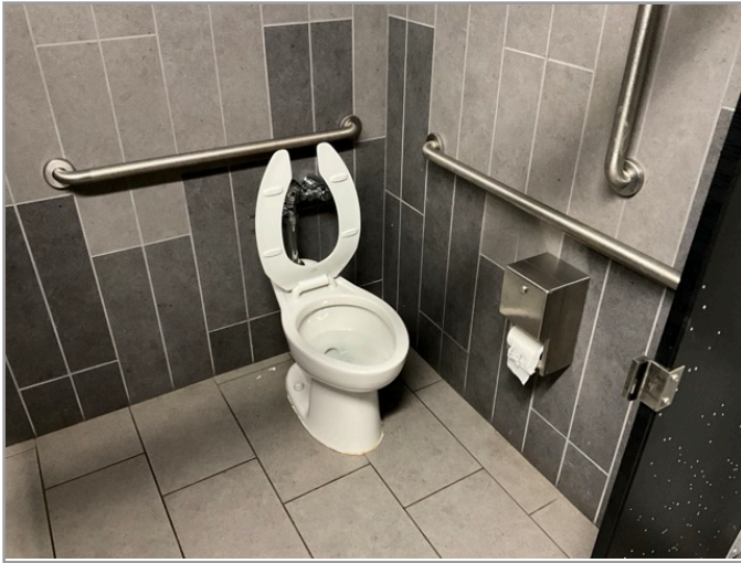
TOILET STALL OVERVIEW
