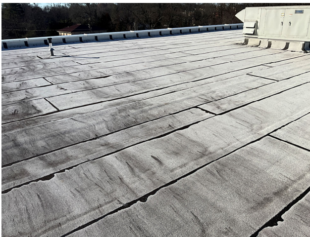
5 - PRIMARY ROOF OVERVIEW
